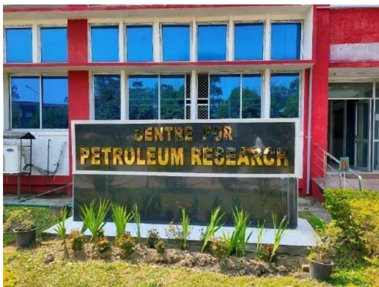
CSIR-NEIST Centre for Petroleum Research
